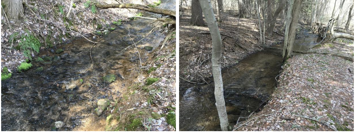
Figure H4. Photographs of the channel connecting the upper and lower reservoirs.
