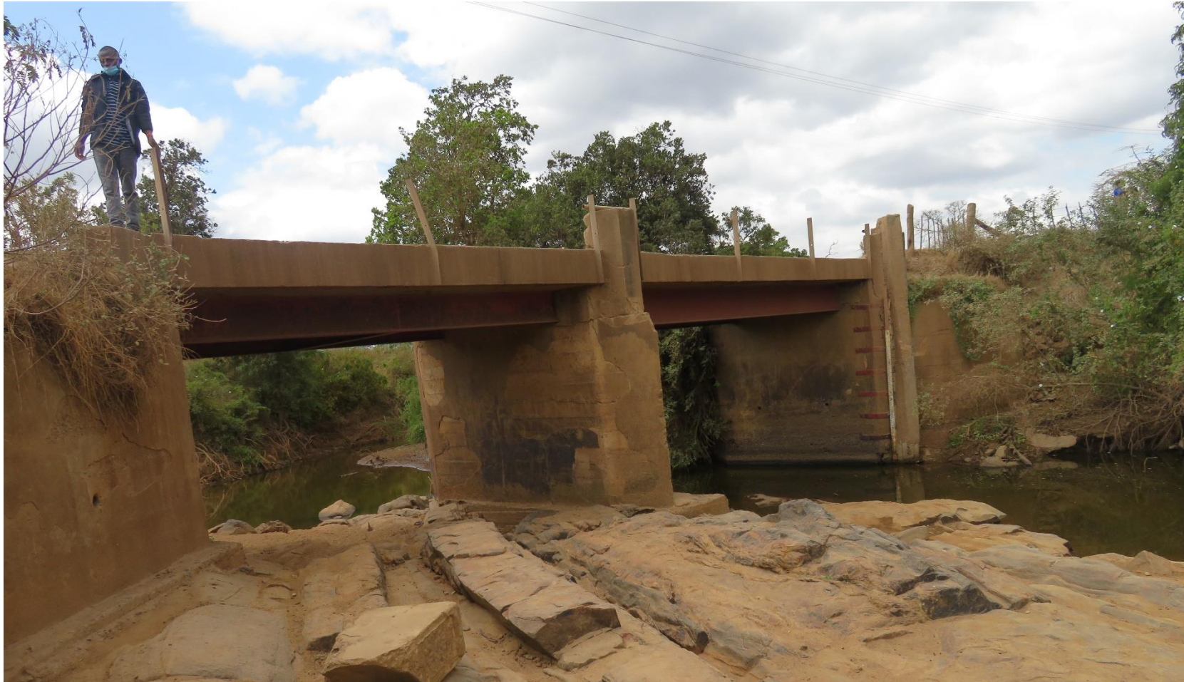
Figure B-7. Doldol – CA07 streamgauge during low/no flow conditions. The stream channel is partially bedrock constricted and the gauge (located to the far right) is located in a pool even when there is no flow. Photo courtesy of author.
