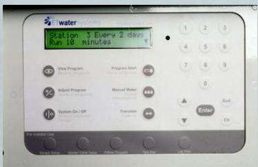
ET Water Smart Controller 100. Signal-based using cellular technology. ASCE method used to calculate ET. Web site used for programming of landscape settings.
