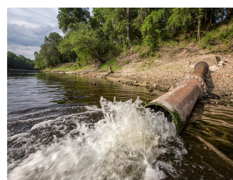
Fig 2: Wastewater discharged into Suwannee river [Credit WJCT News].
