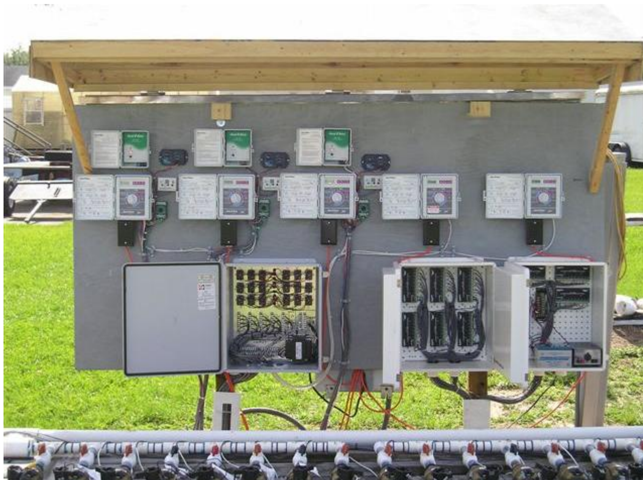
Figure 2-8. Control board showing time clocks, soil moisture sensor-controllers, solenoid valves wiring, and flowmeters data acquisition system (details are shown in the next Figures).
